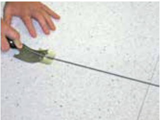
Welding bead is trimmed in two steps, with an initial trim using a trim plate.
