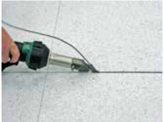
Welding bead is placed in the groove and fused by heat application.
