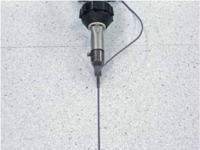
> Welding Beads are .160" (4mm) in size.
